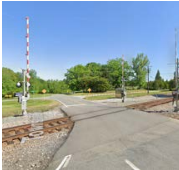
Figure 4 - Norfolk Southern Railway crossing.
