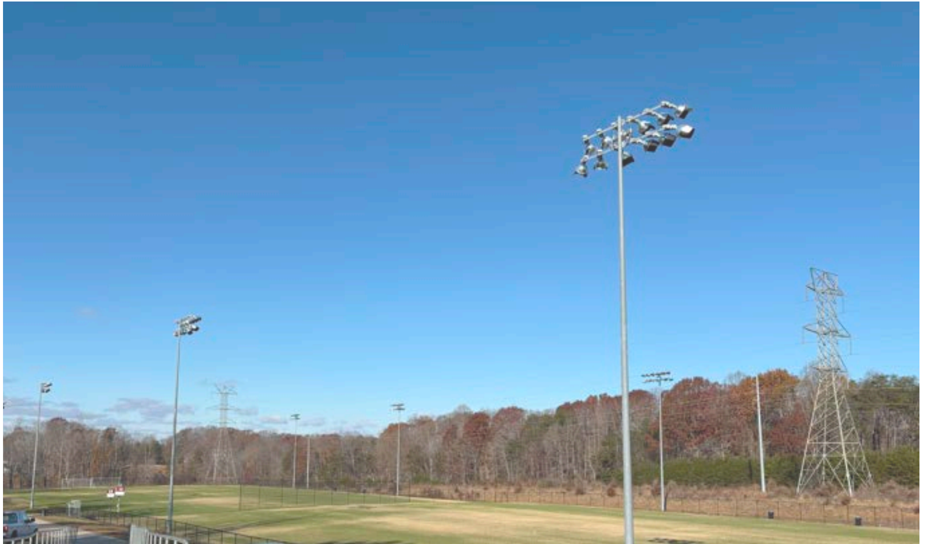
Figure 20 - Image of Duke Power right-of-way and high tension wires north of fields 12 and 13.
