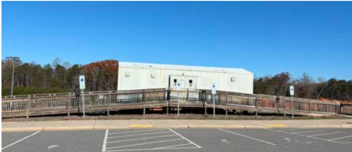
Figure 11 - Temporary mobile restroom facility.
