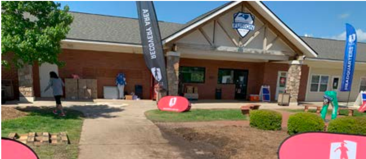
Figure 6 - The Field House.
