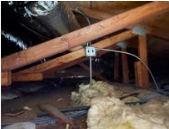
Photo 1 – Attic Wood Roof Trusses
