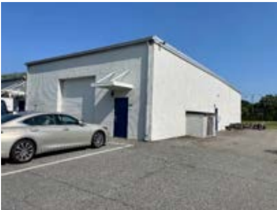
Photo 9 – Exterior Load bearing CMU
