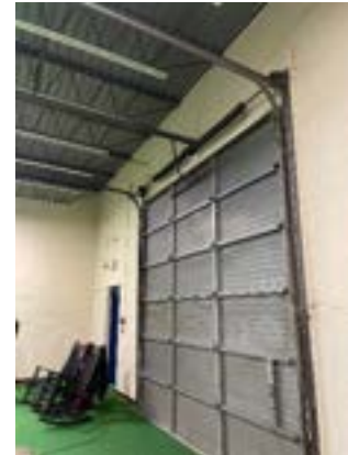
Photo 8 – Exterior Load bearing CMU
