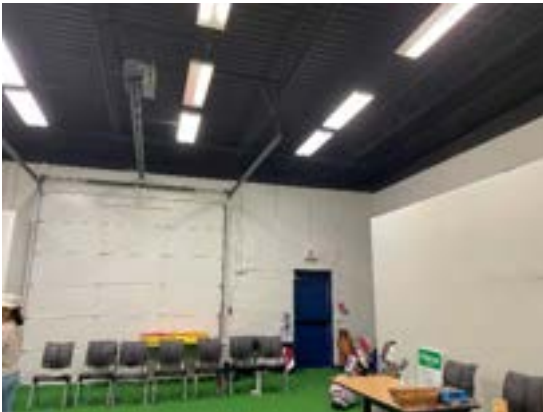
Photo 7 – Roll-up garage doors
