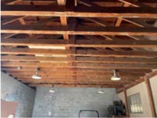
Photo 19 – Wood Roof Trusses
