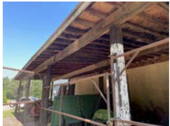
Photo 23 – Wood Framed Canopy
