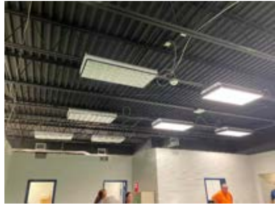
Photo 6 – Steel Bar Joists
