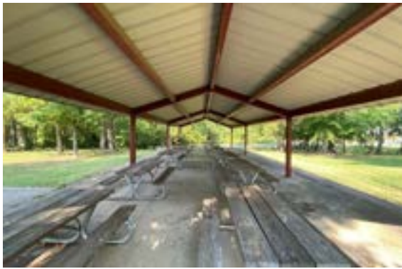
Photo 3 – View of Underside
