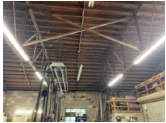
Photo 14 – Steel Truss bracing
