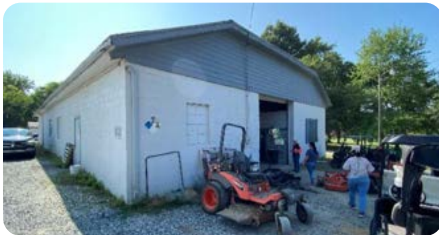
▲ Maintenance Building exterior view
