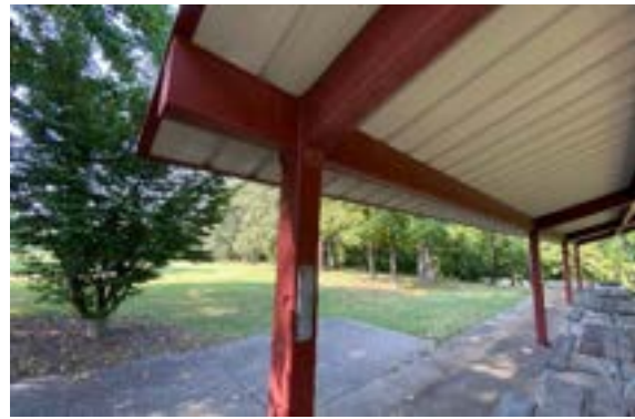
Photo 4 – View of Steel Frame
