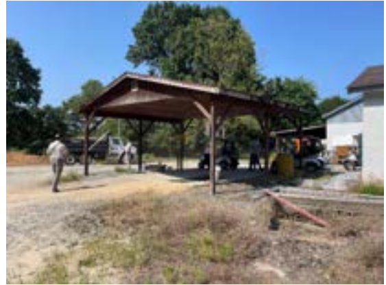
Photo 25 – Wood Framed Maintenance Pavilion
