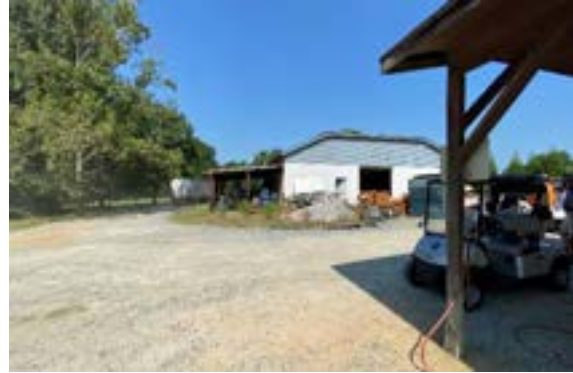
Photo 2 – East Elevation With Covered Area
