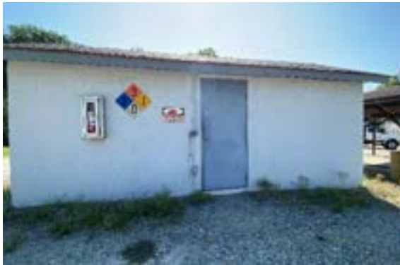
Photo 8 – Maint. – Hazardous Material Shed (not observed)
