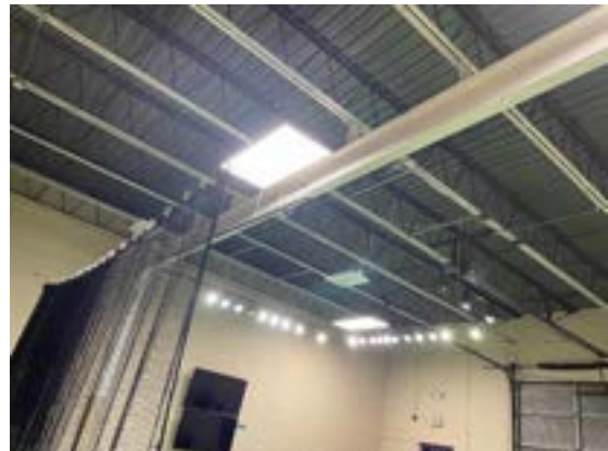
Photo 10 – Service crane rail structure
