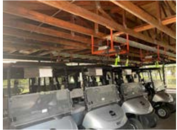
Photo 4 – Wood Roof Trusses
