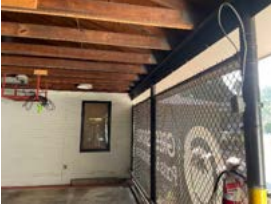
Photo 3 – Wood Roof Trusses & Perimeter Steel Beams
