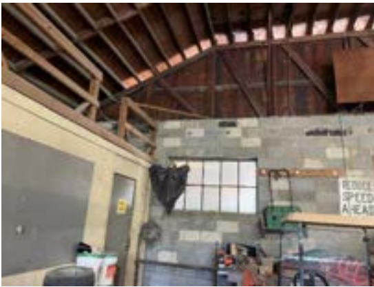
Photo 15 – Office space & mezzanine
