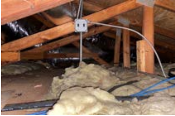
Photo 5 – Attic Access showing trusses & insulation
