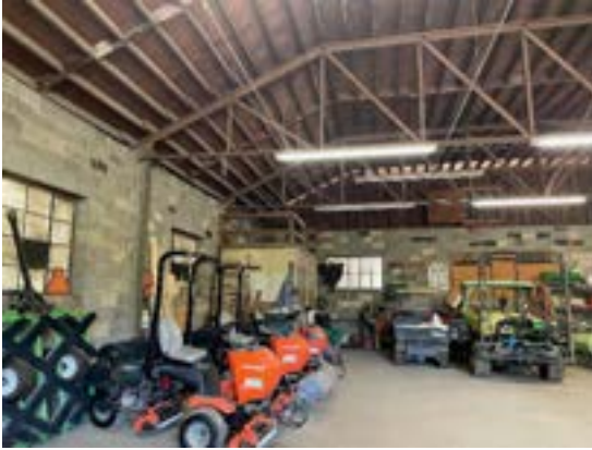
Photo 13 – Steel Truss with wood purlins
