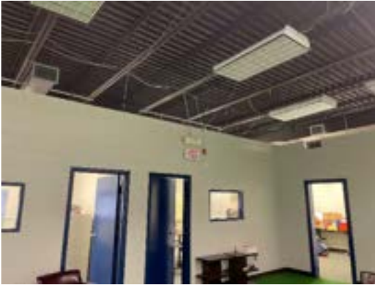
Photo 5 – Steel Bar Joists
