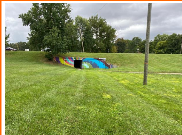
View facing south from near Sounding B-7
